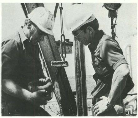
tive at Carlsbad, and Dave Ogden, left, driller for Sonora Drilling Company, examine the diamond bit used for cutting cores. Drilling program consists of coring to depths of 800-plus metres so that the underlying salt beds can be scientifically evaluated. A hydrological study of the area is using separate drill holes to gain data for the calculation of possible radioisotope migration.
